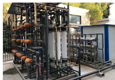
Reclaimed water reuse system
